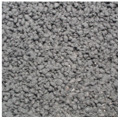
Figure 4.2: Bitumen coverage of aggregate at initial stage
