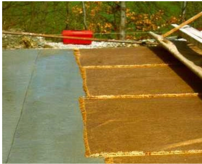
Figure 4.10: Longitudinal structuring of cement concrete with burlap
