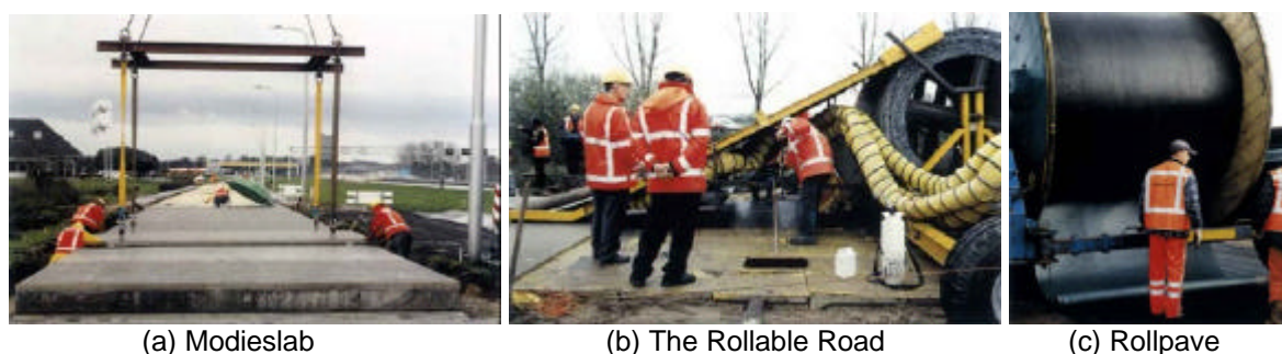
Figure 6.3: Examples of modular road surfaces tested during Dutch "Roads To The Future" project
