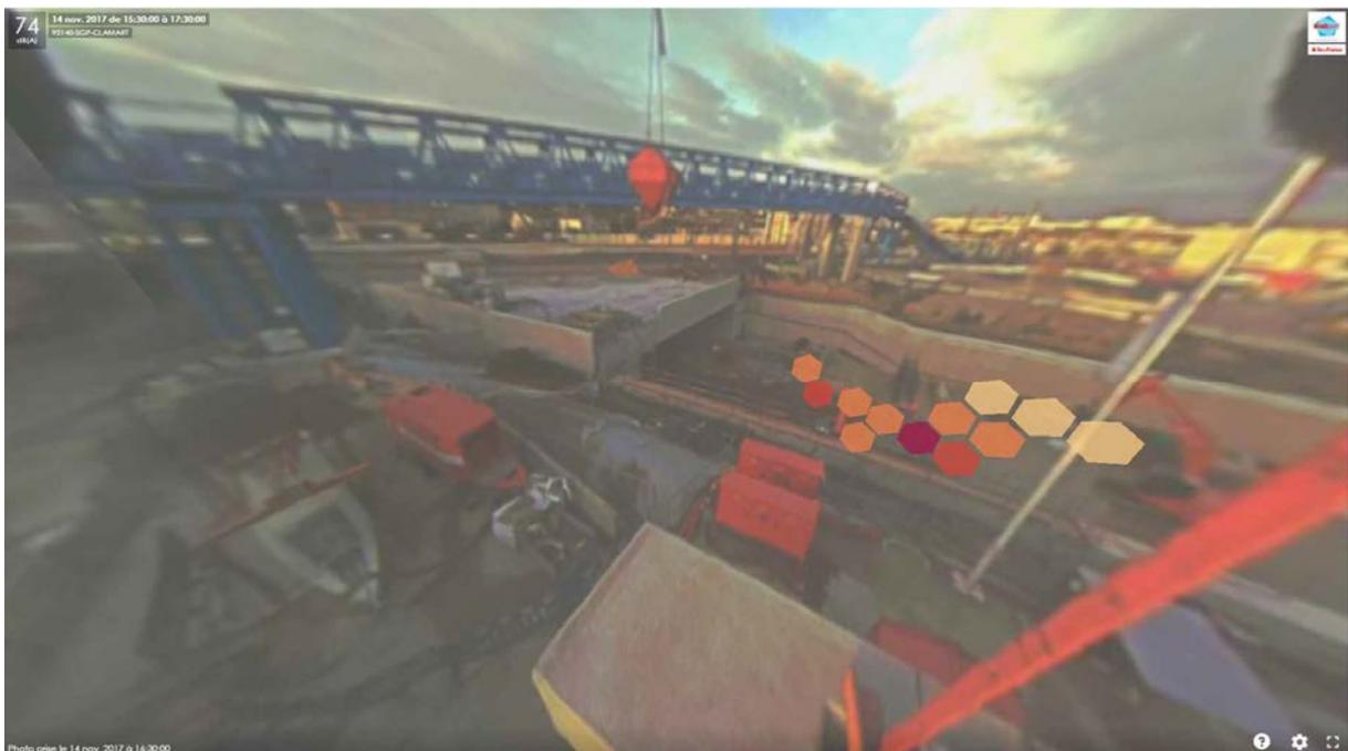
Figure 2: One of the images from one of the "medusa" sensor deployed at the Grand Paris Express construction site in Clamart. It shows that two thirds of the sound energy emitted towards this sensor, during two hours between 15h30 and 17h30 on November 14, 2017, comes from a precise place of the construction site (in red). The noise level observed at the sensor is 74 dB(A).
